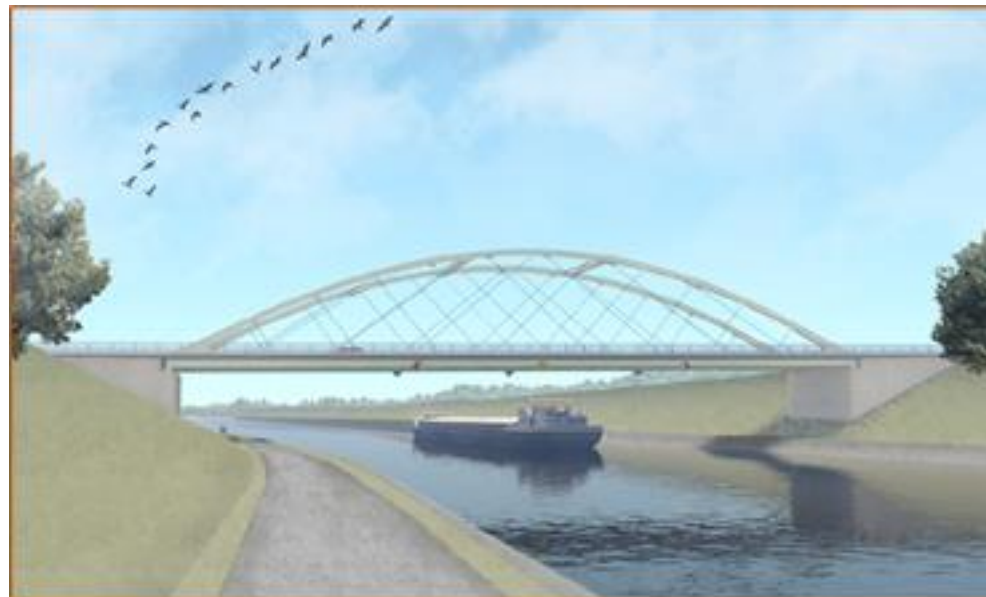
Figure 11 - Ouvrages de type Bow-string (source : ONE 2021)
