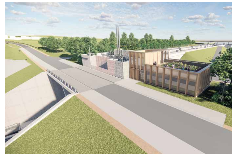
Écluse de Noyon © AEI – ONE-SCSNE
